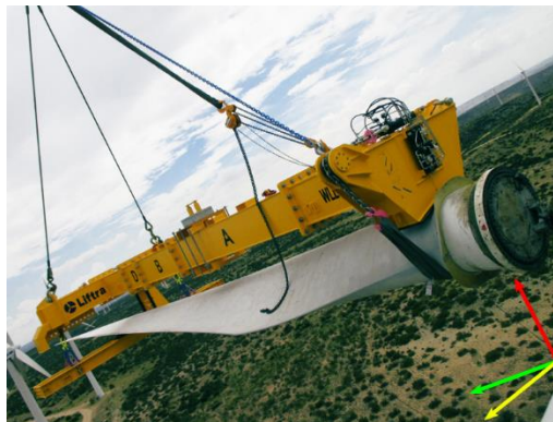
Figure 1: Yoke mechanism with coordinate system X-Y-Z being yellow, red, and green, respectively.
